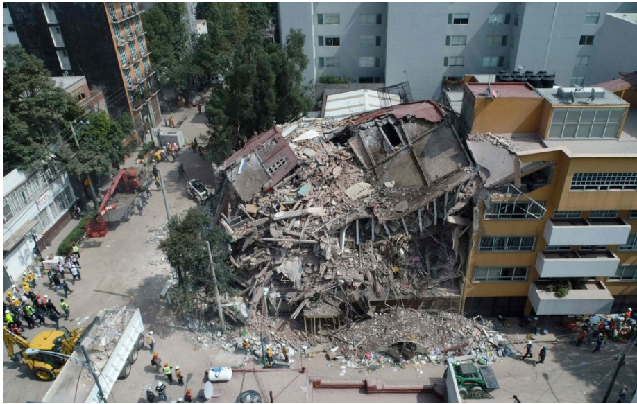
Why Did So Many Buildings Collapse?
